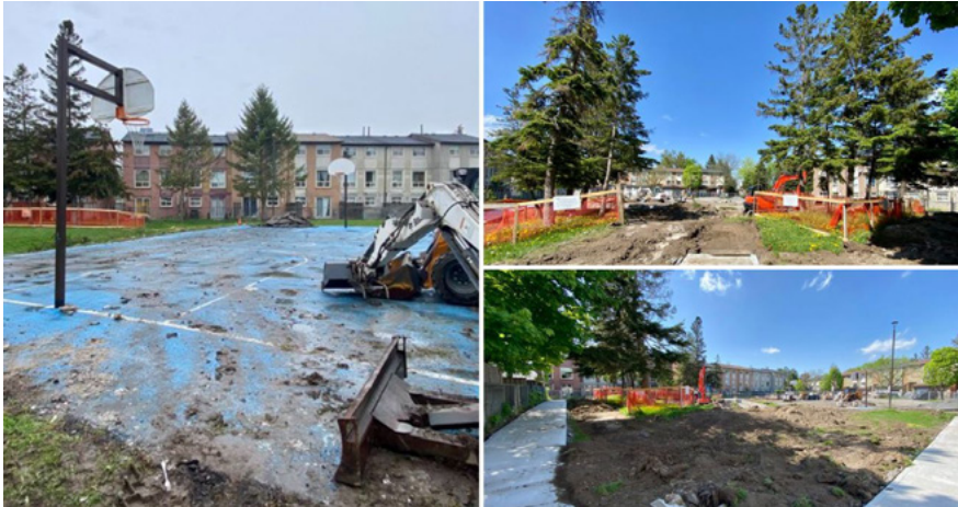
The Empringham basketball court being replaced.
