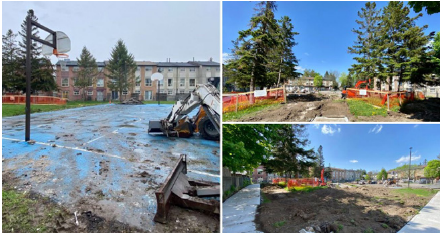
The Empringham basketball court being replaced.
